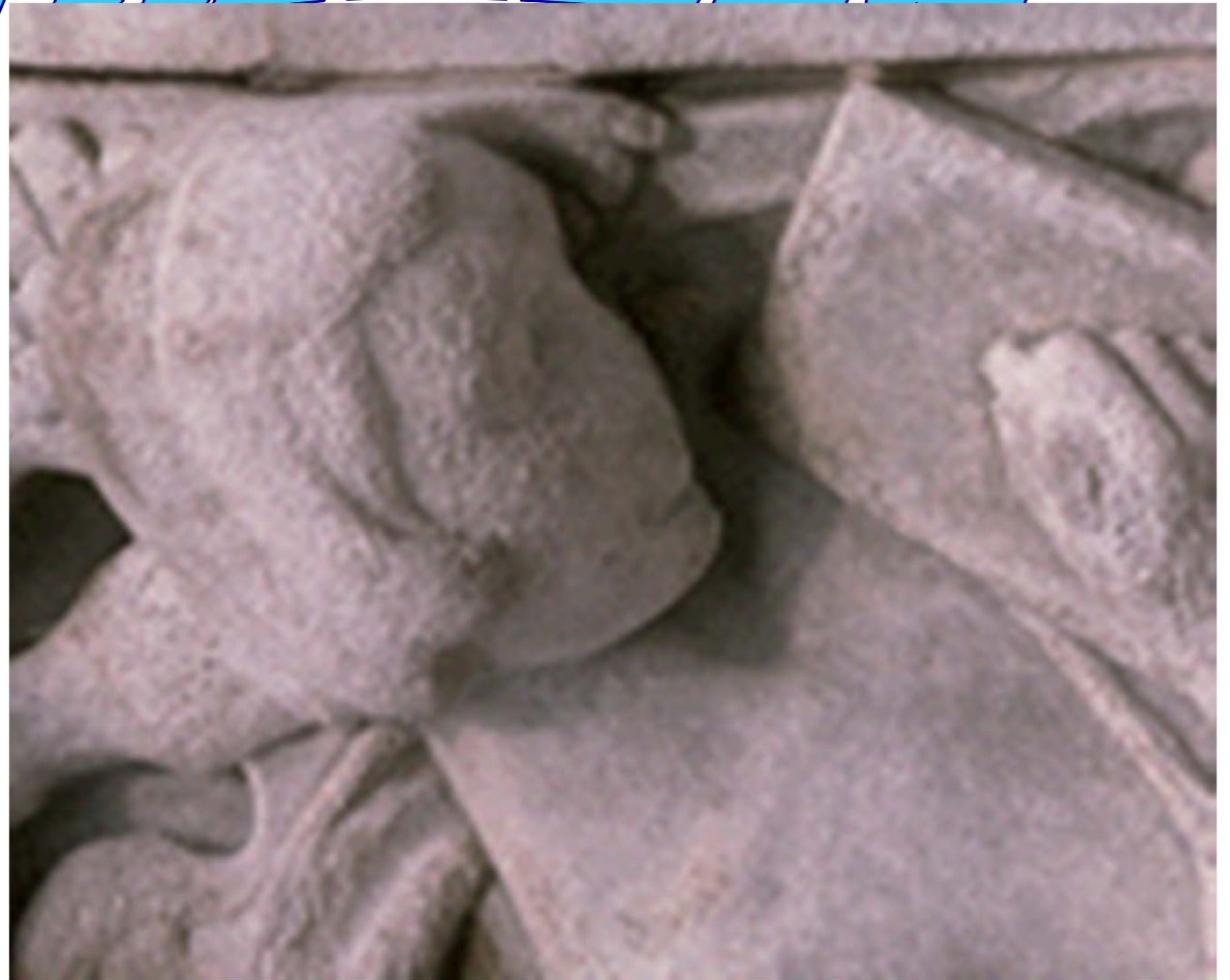
Effects of acid rain on limestone statues and buildings
